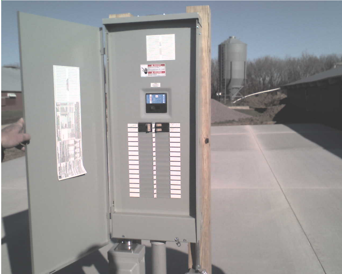
Electric supply installed and concrete pad constructed at site for gasifier system at P & J Products
